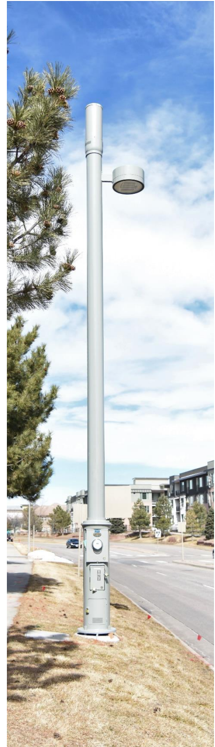
Figure 4-2: Acceptable Combination Pole Installation
