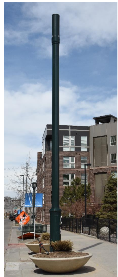
Figure 5-1: Freestanding Small Cell
